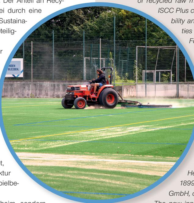
► At TSG 1899 Hoffenheim's junior training center, a pitch based on this recycling technology was installed for the first time in Germany: The artificial turf fibers are made of a polyethylene produced from 100% mixed recycled plastic waste. The proportion of recycled raw material in the fiber is ensured by ISCC Plus certification (International Sustainability and Carbon Certification) of all parties involved in the supply chain.
